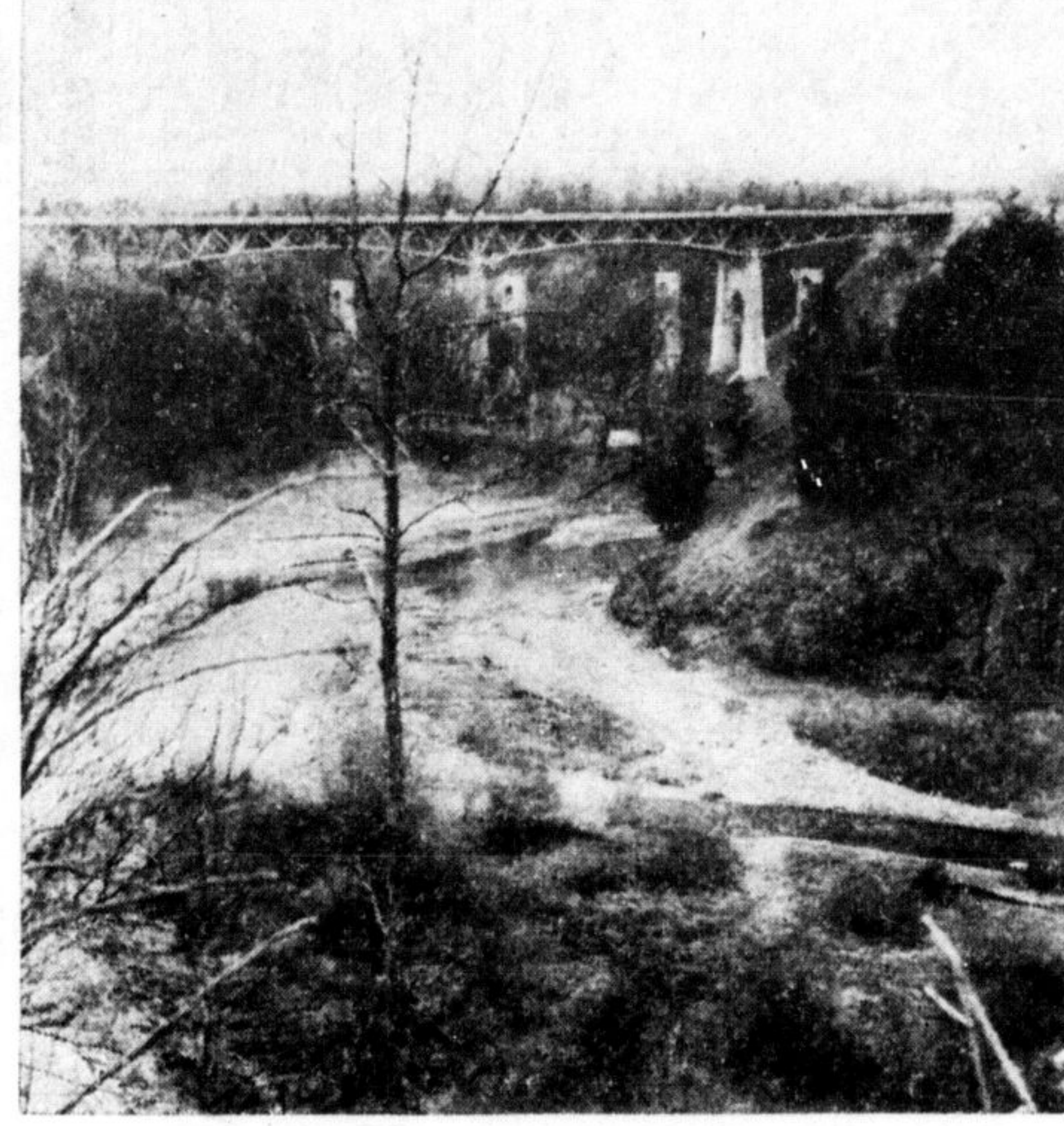
LOOKING TOWARD TANSLEY BRIDGE FROM VALLEY Note columns from the old bridge below
