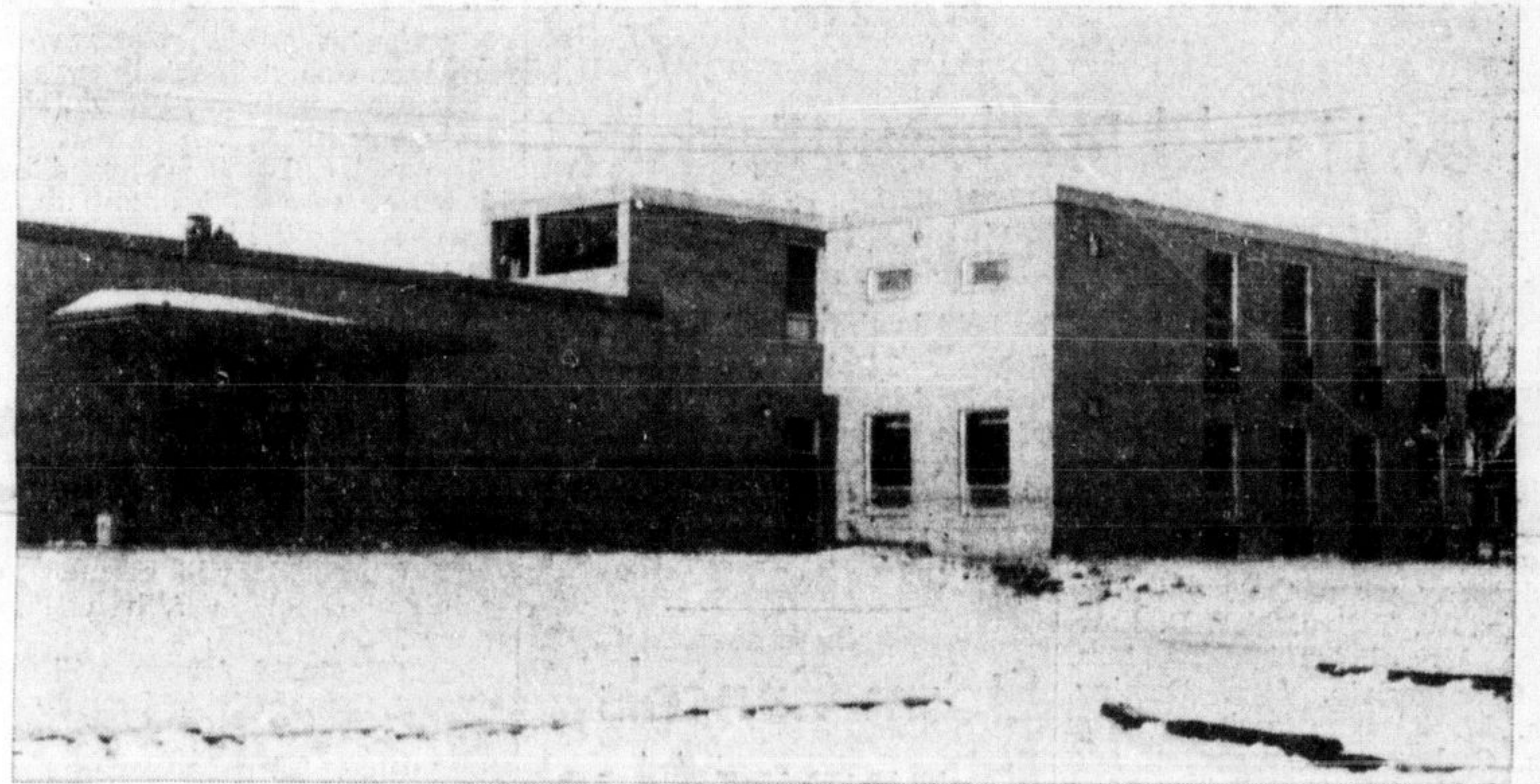
THE NEW $80,000 ADDITION at Holy Rosary Separate school will be officially opened and dedicated by Bishop J. F. Ryan on Sunday afternoon, in a 2.30 p.m. ceremony at the Martin St. school. The four-room addition brings the school up to 14 rooms. The addition is the two-storey section shown at the right of this picture, with two classrooms on the ground level, and two classrooms upstairs. It branches out from the north rear corner of the school.
