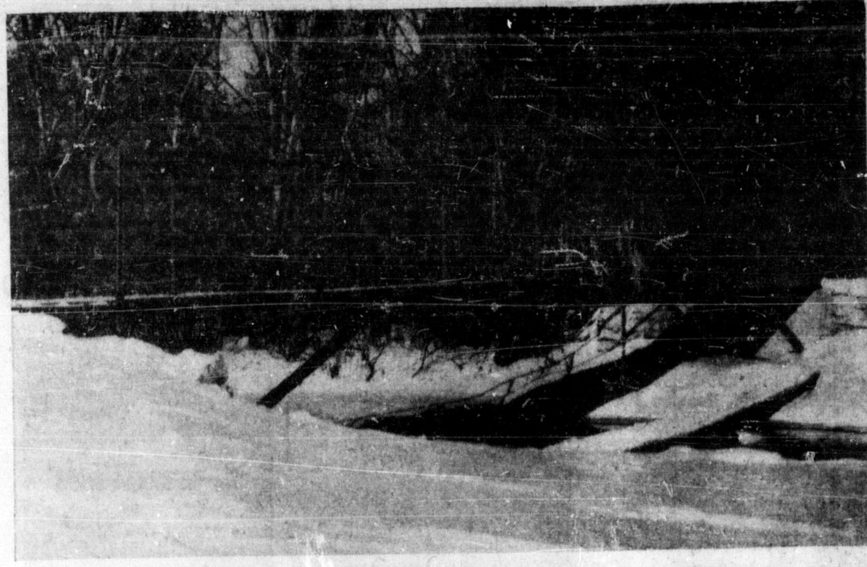
PARKWAY FOOTBRIDGE CROSSES SIXTEEN
