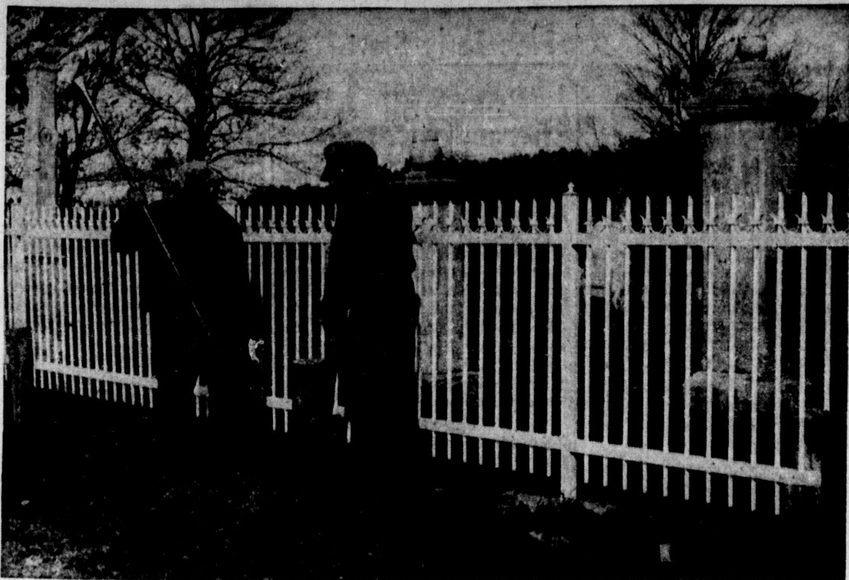
THE PIONEER CEMETERY boasts a fine looking fence these days, following many hours of work by the town works department. This summer complaints were registered about the rusty fence which was falling down at the Bronte St. cemetery, and the town was urged to clean up the property where the town's pioneers rest. Workmen took down the fence, had it repaired white, and cemented the posts in. Above, Bill Fetter and Ed Mosley work on posts and cables which will keep cars from hitting the fence.
