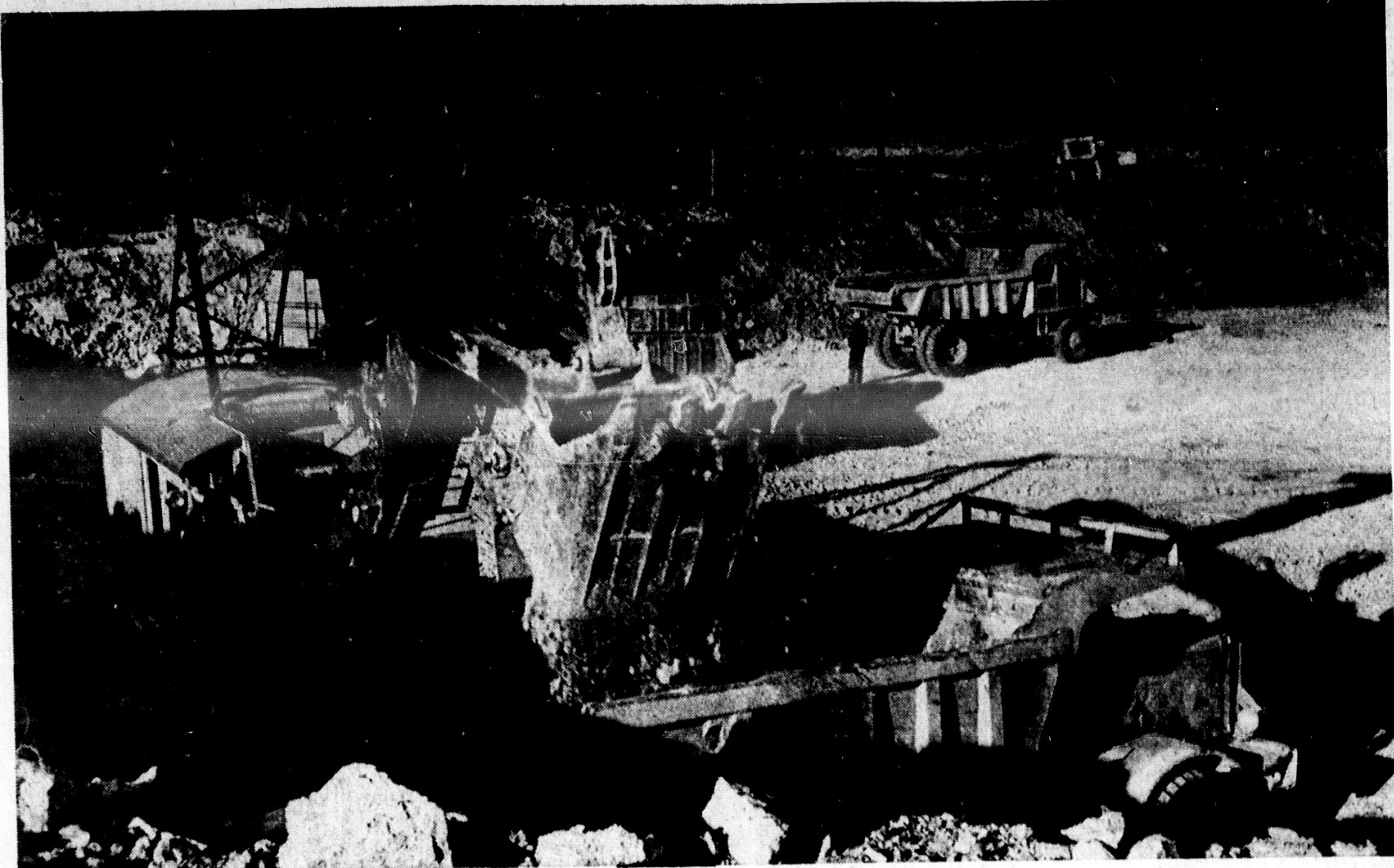
SCOOPING UP THE ROCK previously blasted out by tons of dynamite, two huge shovels are engaged in cutting the path of Highway 401 through western Halton County. Here, the shovels load two of the five Euclid trucks which are carrying away the rock to form a fill base for the road on another section of the mid-Halton route. The new highway cuts over and under concession lines, through fields and the occasional home as it makes a path throughout the province.
