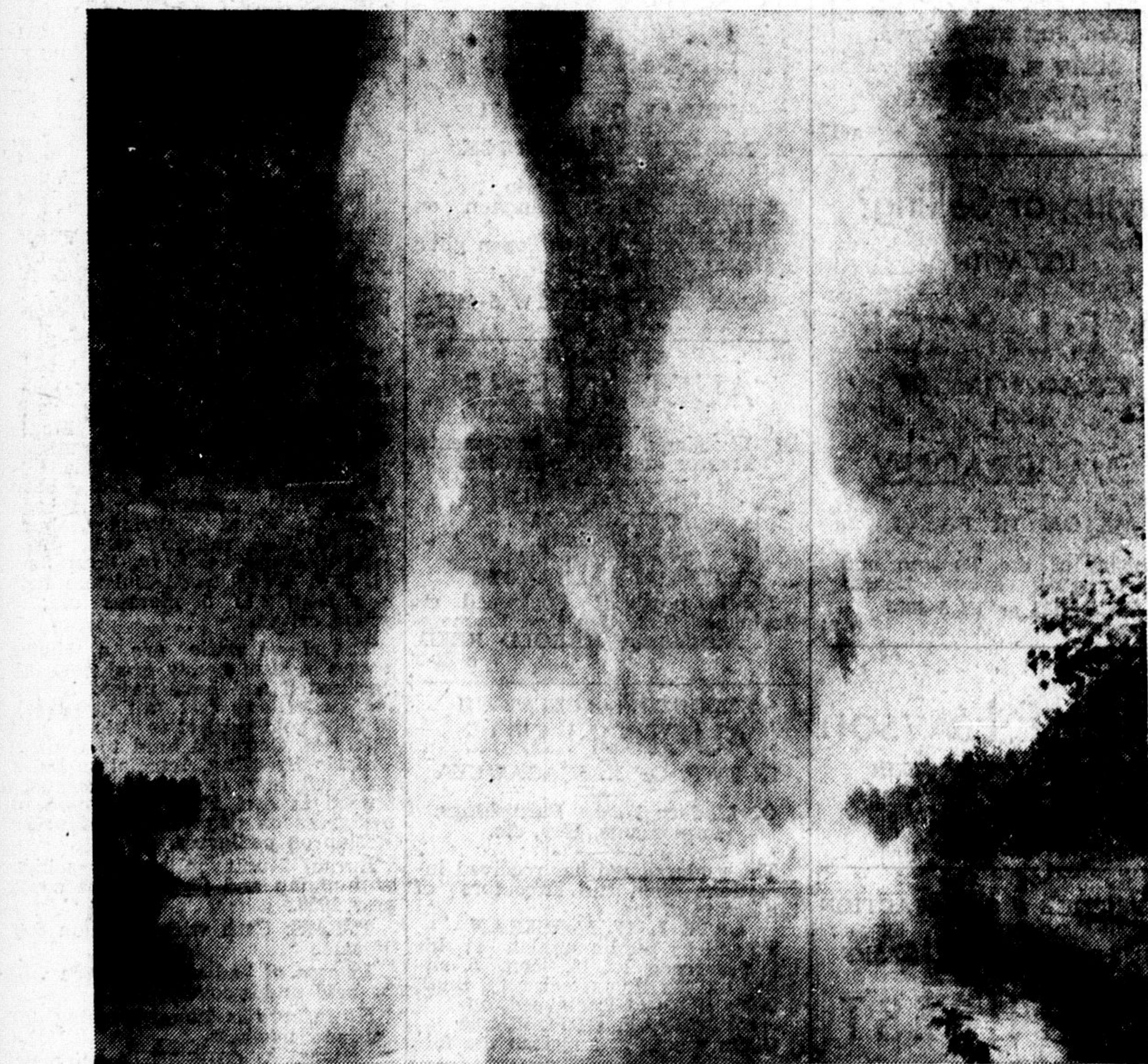
THIS BLAST at the Ground Hog river used about 14,000 pounds of a type of dynamite (Hi-Velocity 60 per cent gelatin) with special underwater detonating qualities to provide a 460-foot long trench, eight feet deep and eight feet wide, in the bed of the river.
