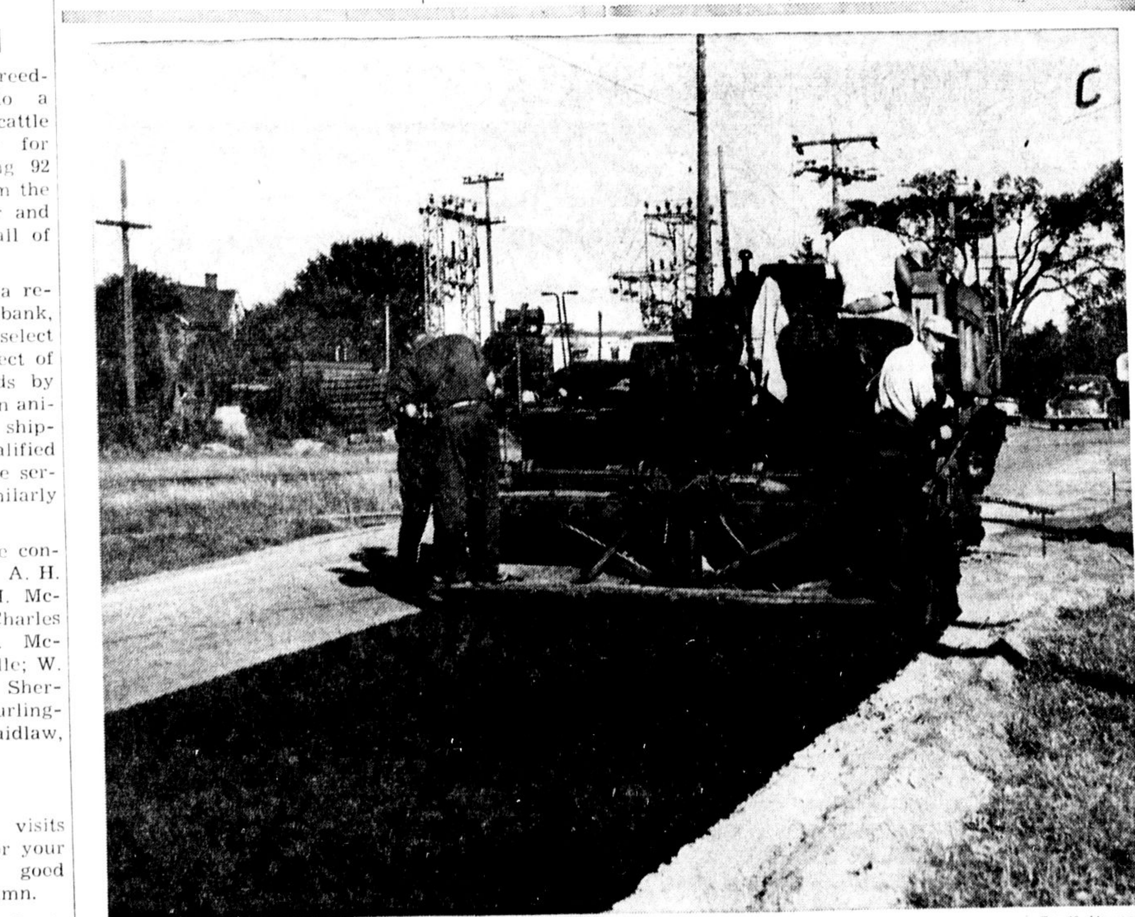
BRONTE STREET IS NOW PAVED from the C.N.R. tracks to No. 10 sideroad, and police are watching the new stretch of excellent road for speeders who might take advantage of it. The King Paving Co. of Oakville did the work for the County of Halton, and shown above, the tarvia machine lays the new covering near the P. L. Robertson plant.
