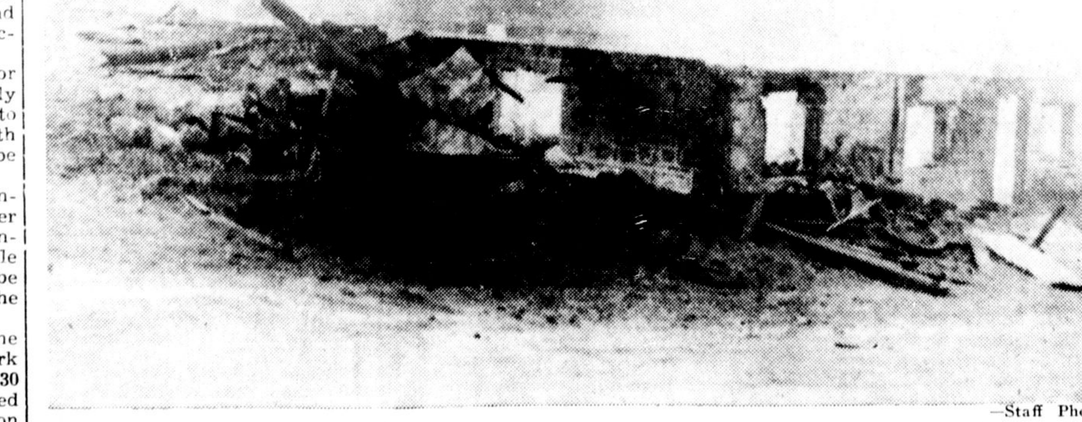
LIGHTNING STRUCK the barn of Peter Patterson, three miles north of Campbellville on the Guelph Road at about 11 p.m. Monday night and the blaze levelled the barn. Damage was estimated between $10,000 and $12,000, partially covered by insurance. The ruins are shown here Tuesday morning still smoking. Nearby buildings were saved through the efforts of the Milton Fire Brigade.
