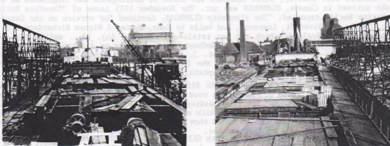
Photos courtesy Don Boone show GLENROSS being lengthened, winter 1925-1926.
