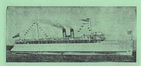
The steamers "Ontario No. 1" and "Ontario No. 2" are of twin-screw, triple expansion, steel construction, with 57 foot beam and 328 foot length. Promenade deck for sports and dancing, and passenger deck with staterooms, parlors, dining salon, and lunch counter.
