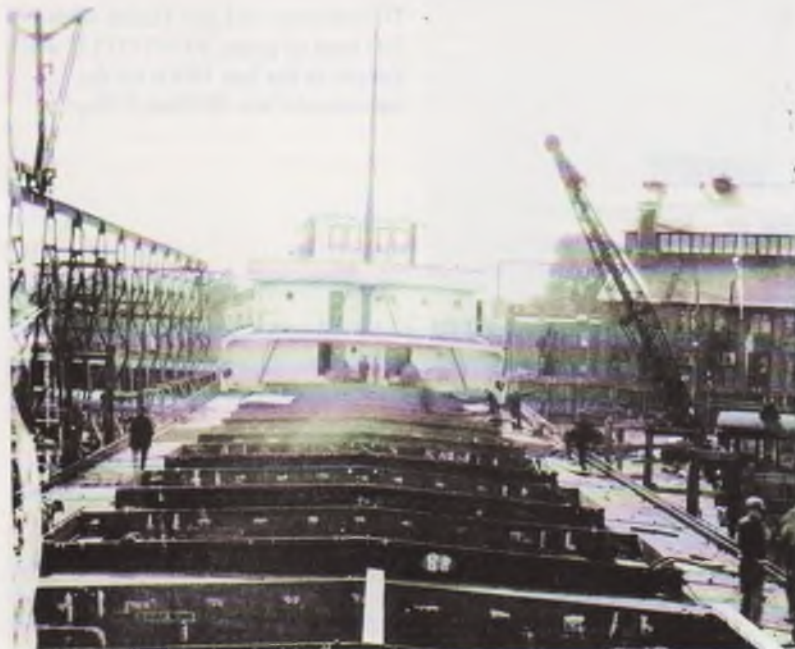
It is Sept. 30, 1925, and the work of lengthening GLENLEDI progresses at Collingwood. Photo courtesy Don Boone.
