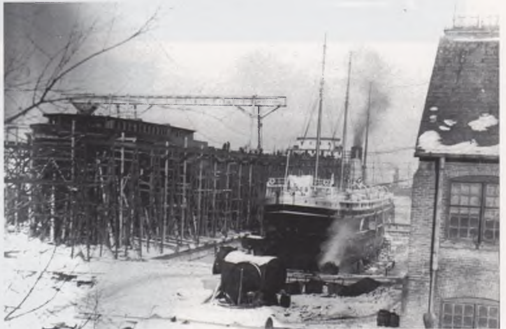
MANITOBA is on the Collingwood drydock in December, 1910. Under construction is the bulk carrier EMPEROR.
