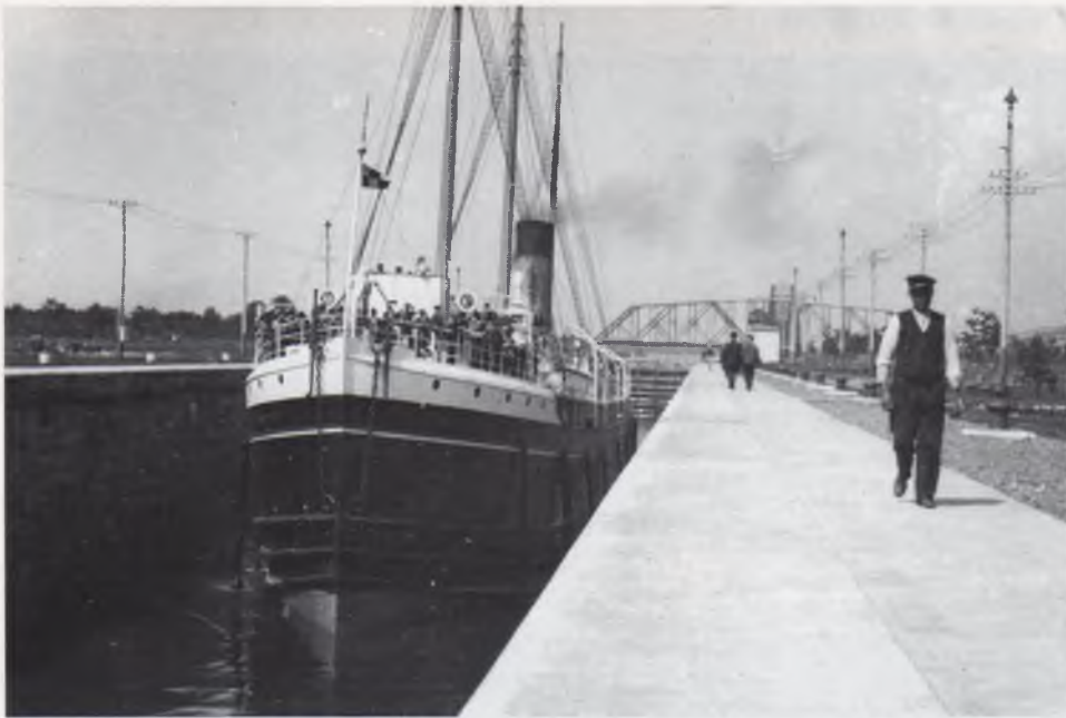
Photo by John Boyd caught MANITOBA in the Canadian Soo Lock in 1908. Note the turtlebacked forecastle.
