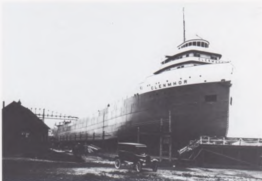
GLENMHOR is on the ways at Midland shortly before her June 23, 1926 launch as GLENMOHR. Photo by J. W. Bald, courtesy Ron Beaupre.
