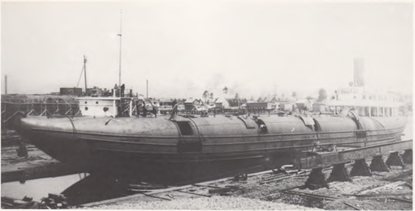
PILLSBURY nears completion in an 1892 photo, courtesy Ken Thro. Note the cargo ports in her side for access to the 'tween deck.
