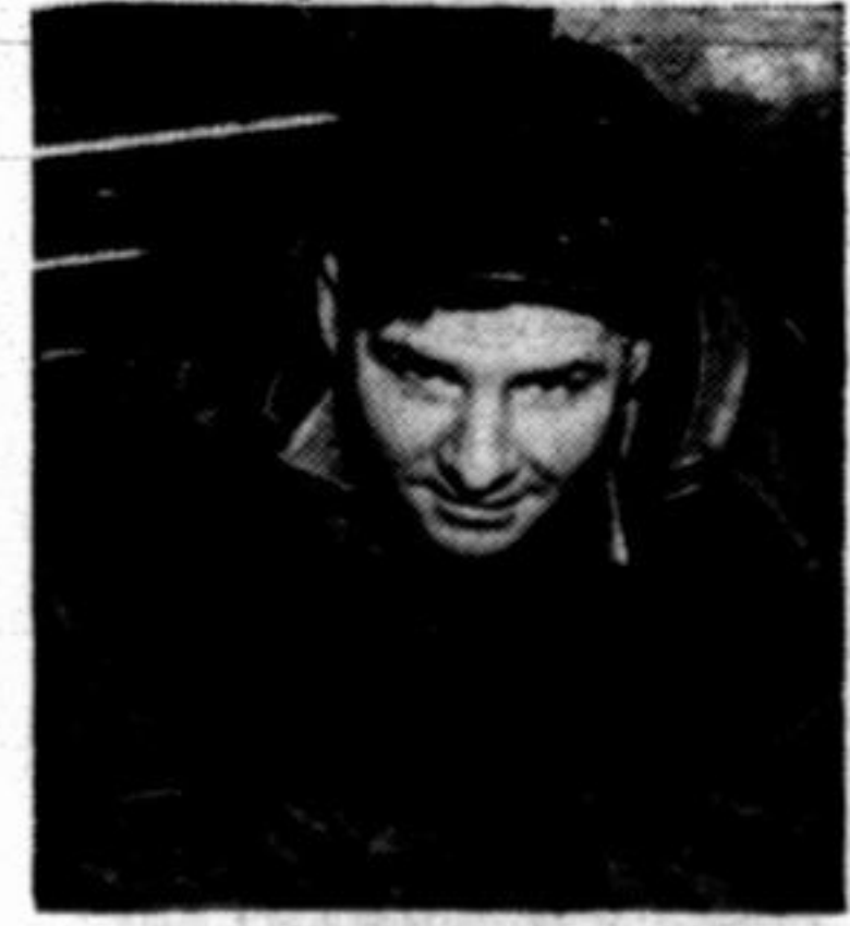
Charles Peters splices cable in the Joliet district.
