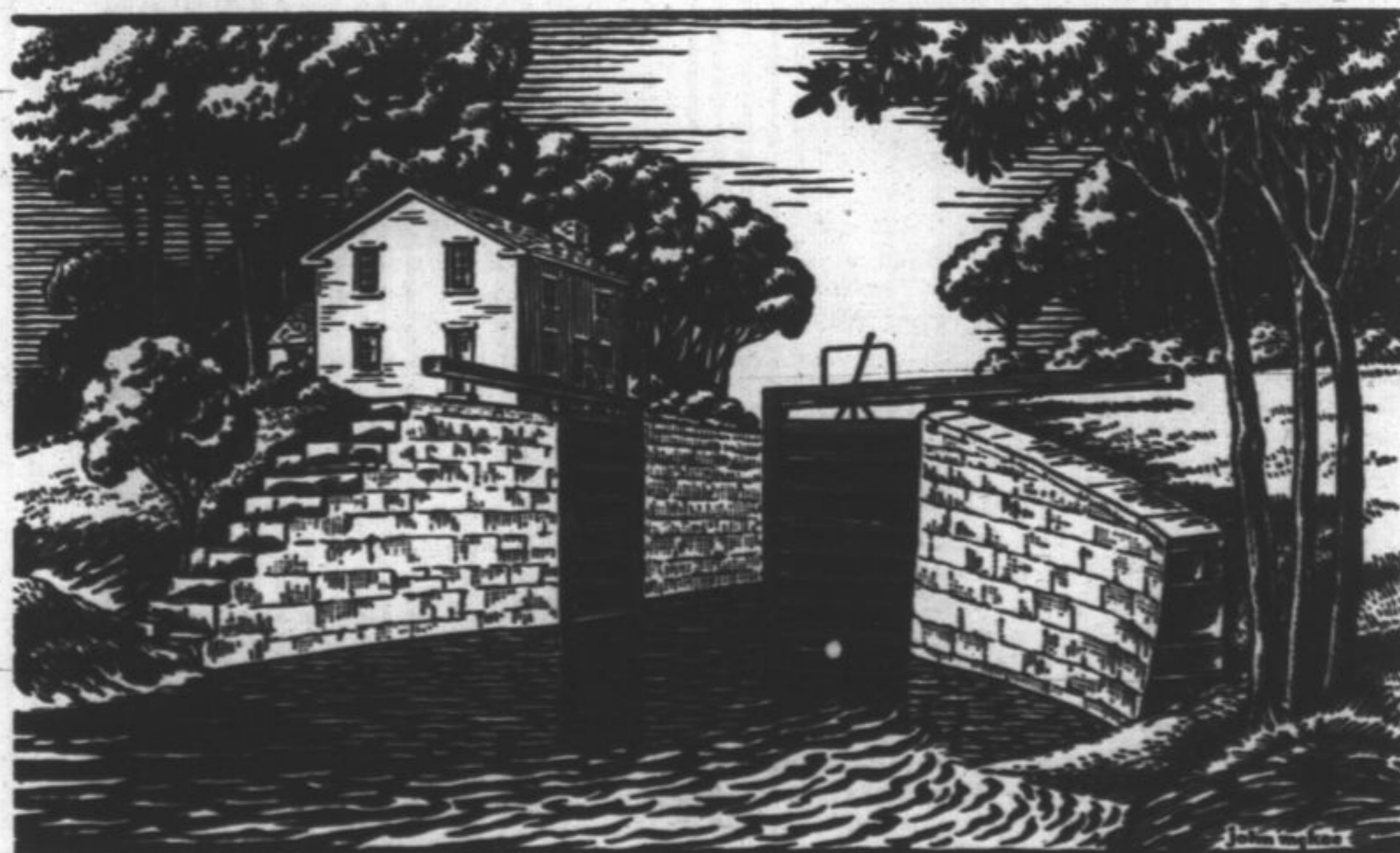
LOCK NO. 6 ON THE ILLINOIS AND MICHIGAN CANAL at CHANNAHON
