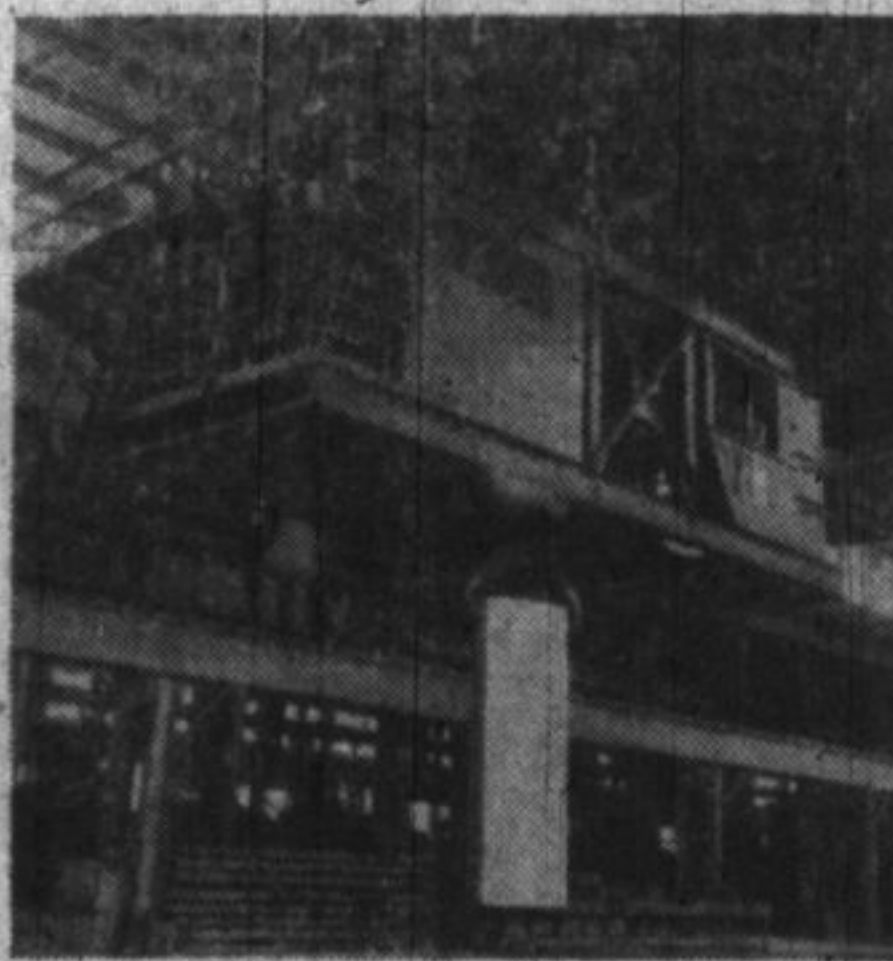
A huge crane, operated by Electric Power, picks up and carries the aluminum ingot to the "continuous" rolling mill. The ingot will be rolled into aircraft sheet.
