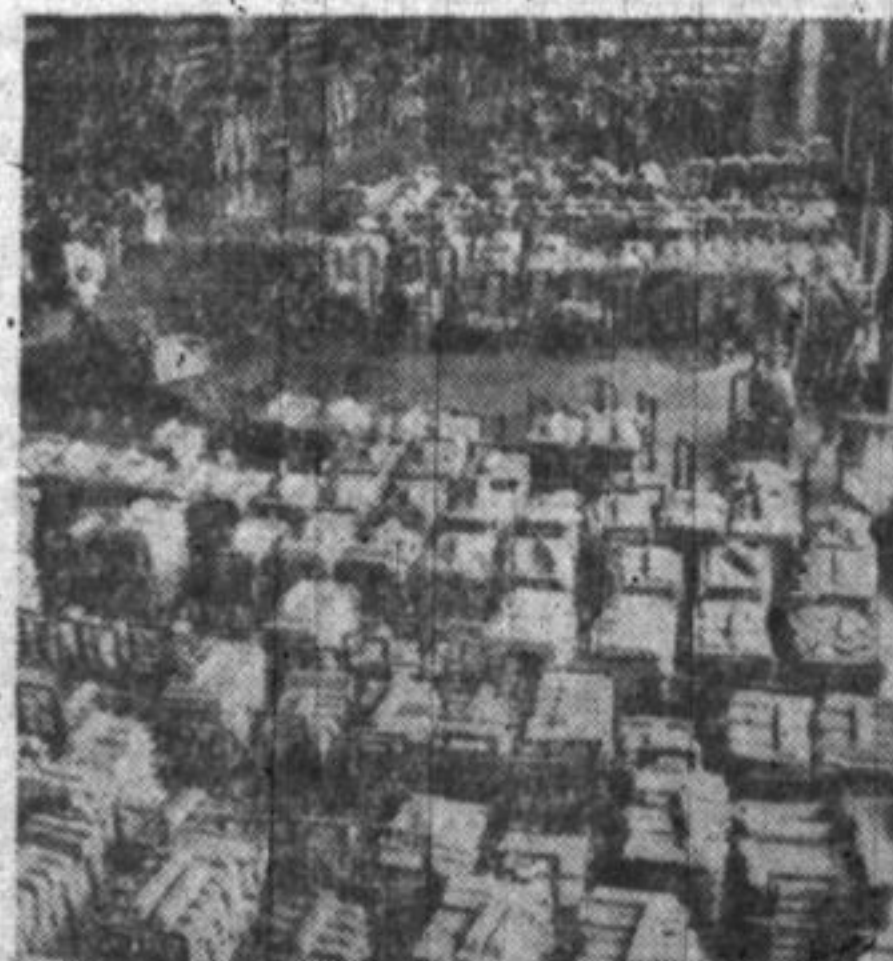
Aluminum pigs in the receiving room of one of the world's largest rolling mills, located in Northern Illinois. In the background are the furnaces where the pigs are melted and combined with other metals for casting into huge ingots.
