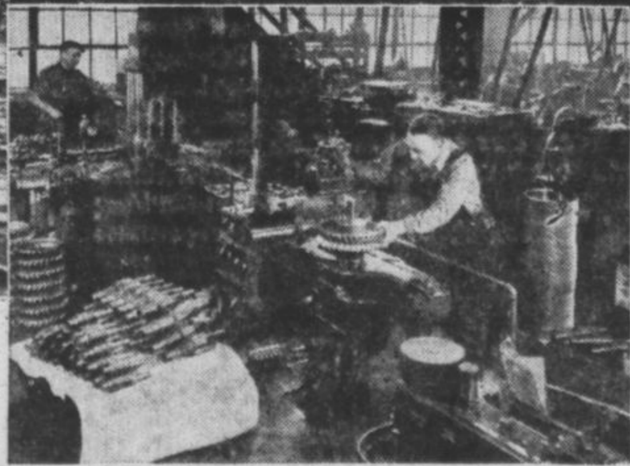
In this Northern Illinois war factory, Electric Power helps produce vital gears for the motors of P-T Boats.
