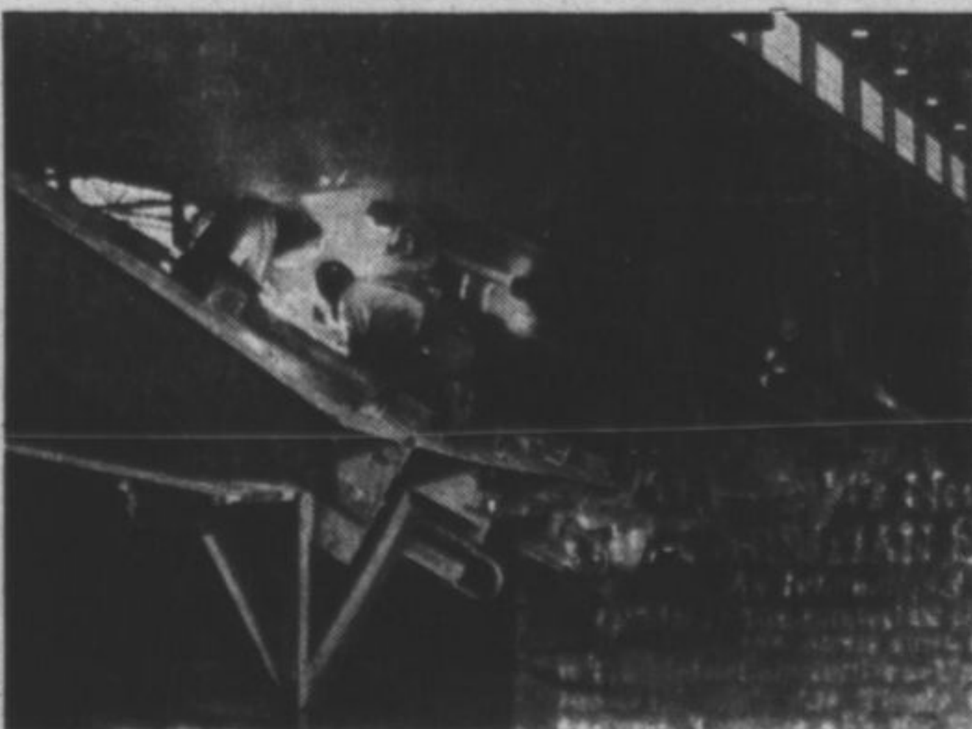
At another ship building plant in the Chicago area a Naval Patrol Vessel is built in sections which are fitted and welded together.
