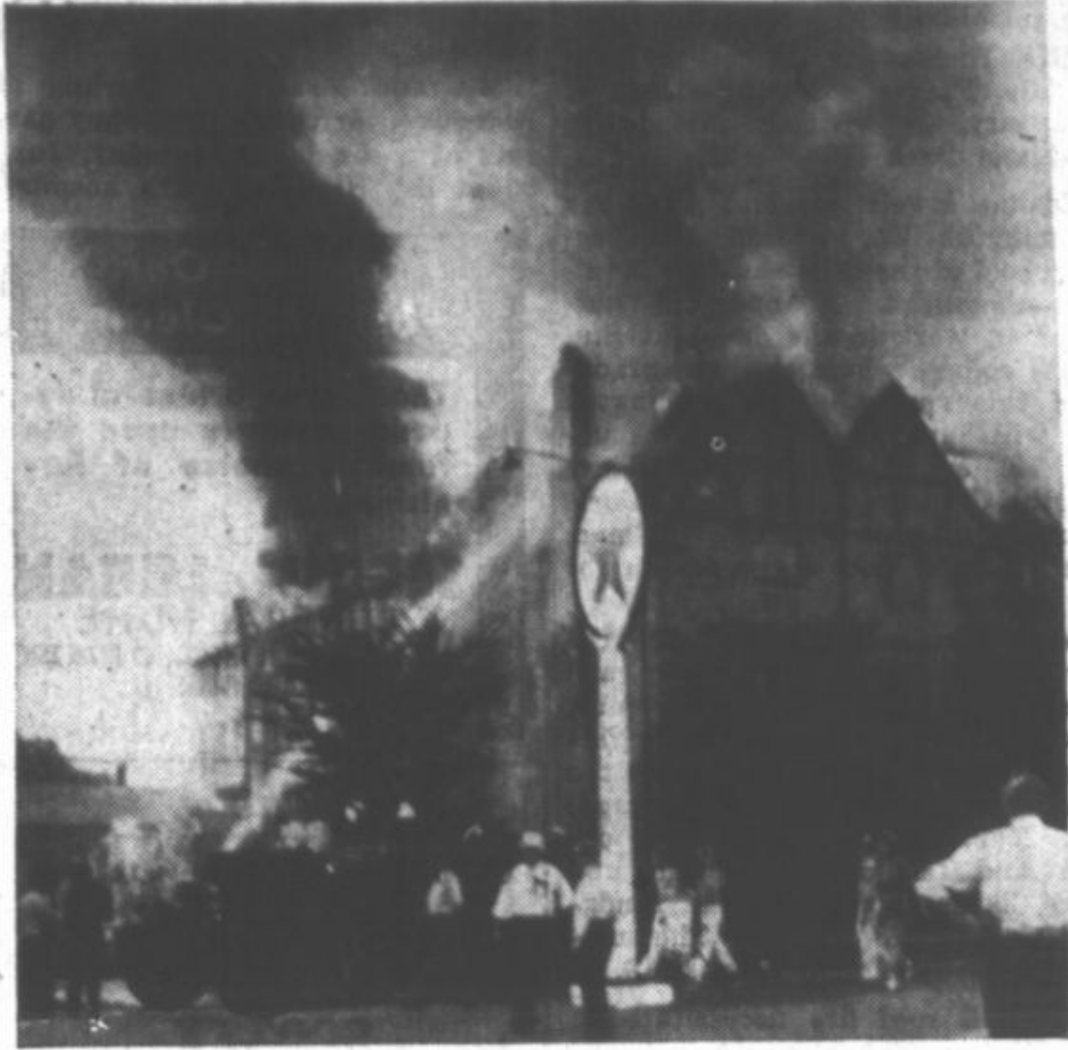
This picture was taken just after the cave-in of the east roof of the Deerpath Inn, in the blaze which caused an estimated damage of $300,000 to the hostelry Wednesday morning.
