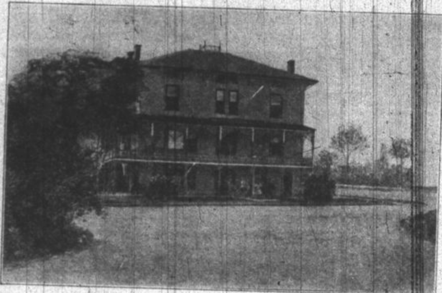
Built in 1852 on the southwest corner of Central Avenue and First Street.
