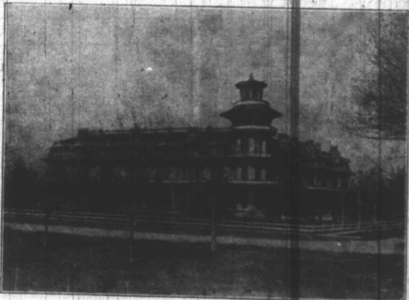
Formerly located at the corner of St. Johns Avenue and Ravine Drive.
