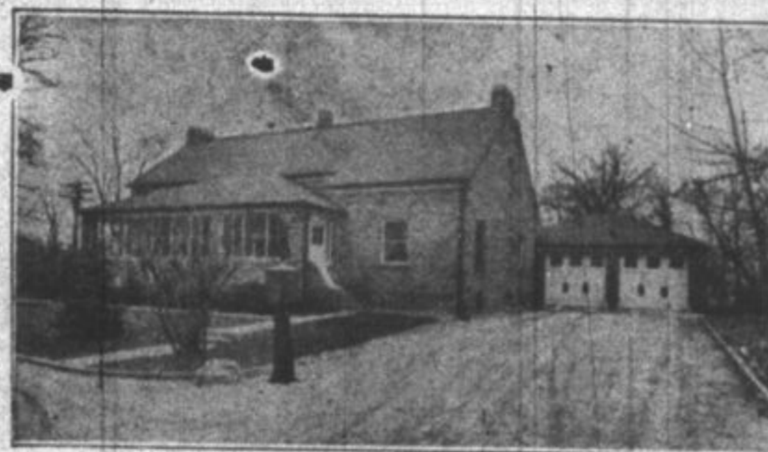
Here is the gas heated home of A. C. C. Timm, Deerfield, Ill., who writes his praise of gas heat as follows:
