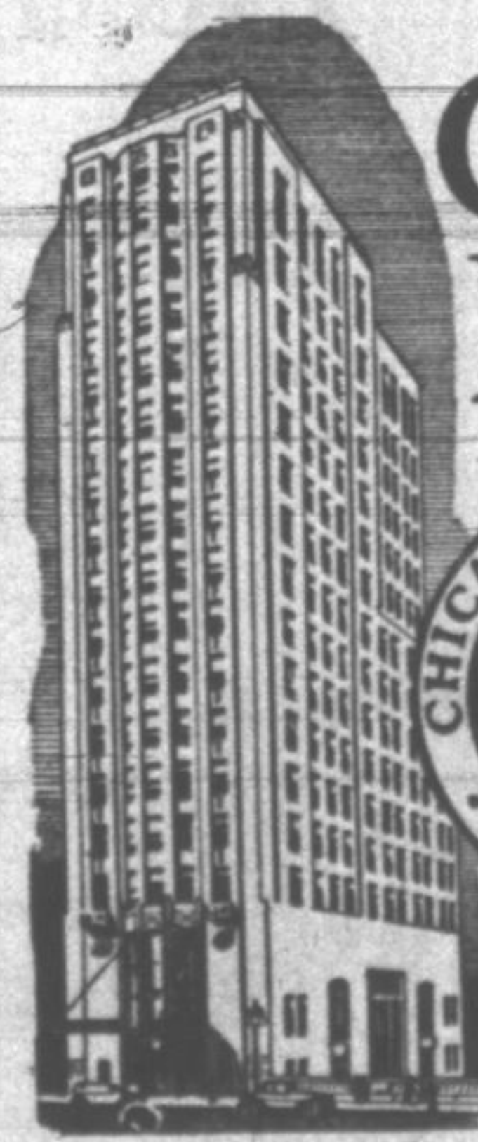
The Chicago Motor Club Building at 66 East South Water Street
