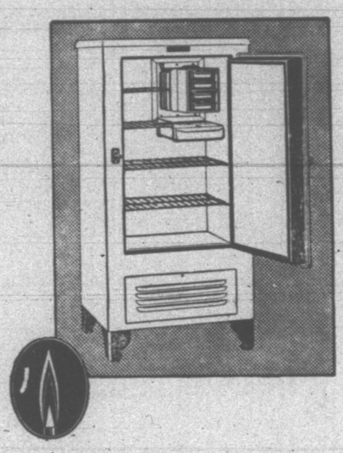
No matter how long you search and shop, you will not find another automatic refrigerator as SILENT as Electrolux. This is no exaggerated claim. The reason is amazingly simple: Electrolux is the only automatic refrigerator operated without the use of machinery. Because of this, it never makes a sound! What's more, it cannot wear out. Moving parts are not included in its cold producing "mechanism." A tiny gas flame and the smallest trickle of water do the work of complicated machinery.
