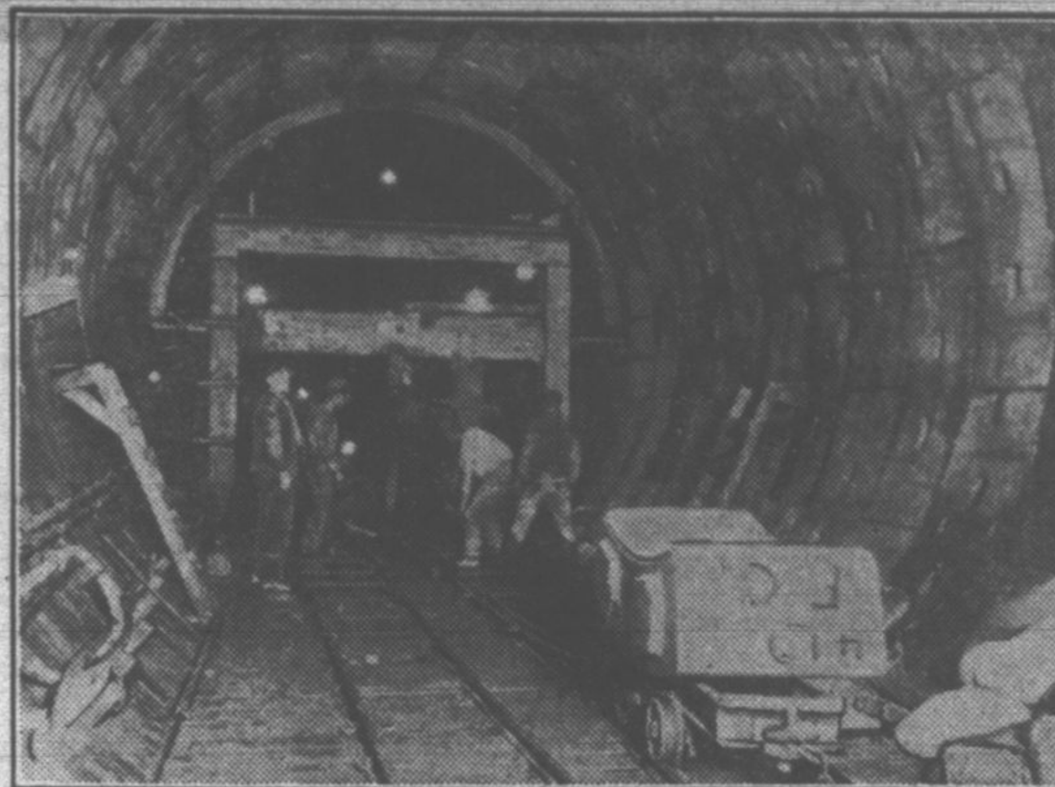
The head of one of the sections of the Ford tunnel showing the machinery used to burrow through the ground. In the foreground is one of the concrete blocks used to line the tunnel which has an inside diameter of fifteen feet.
