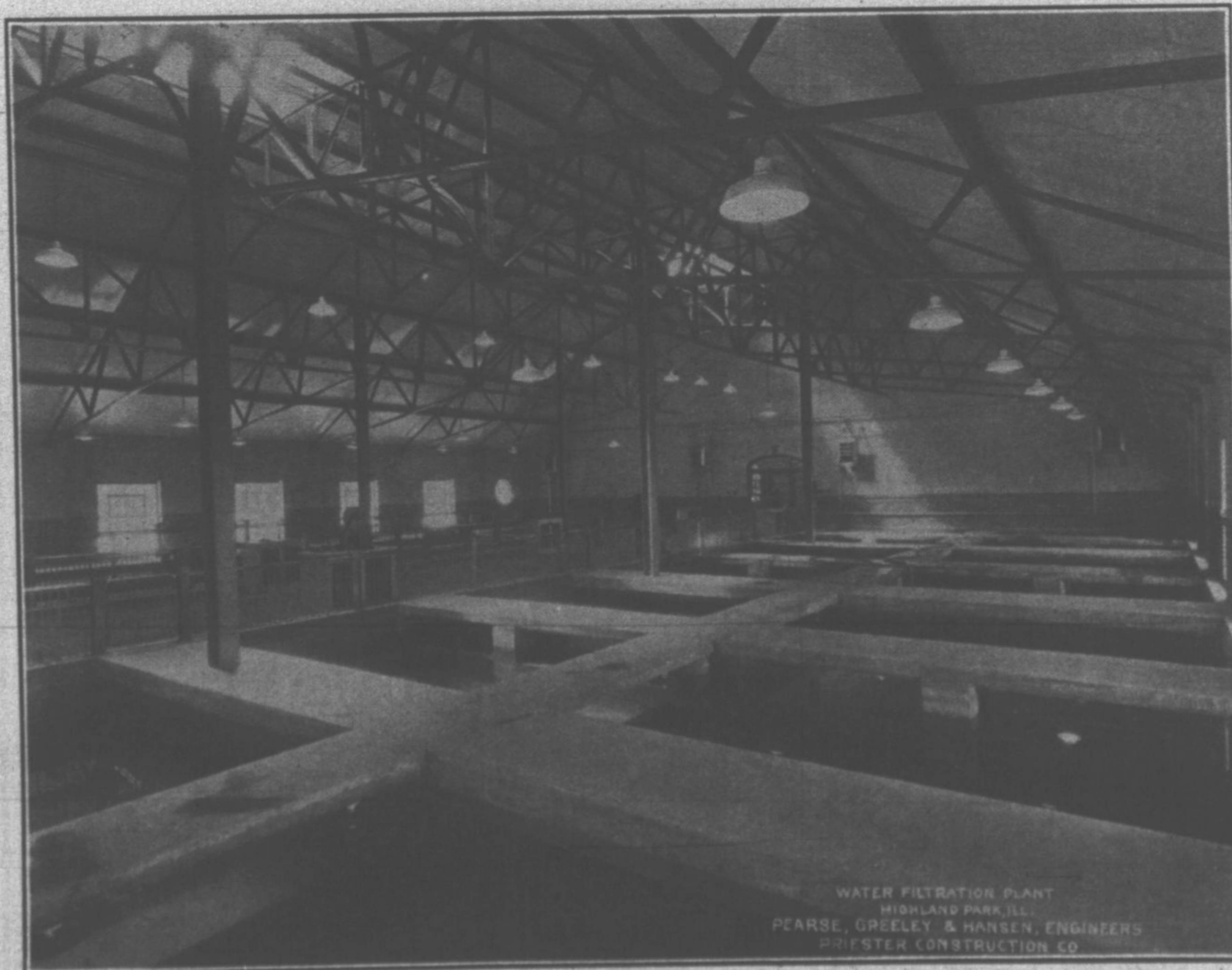
A picture of the Filter Room with the Filter Beds in the foreground
