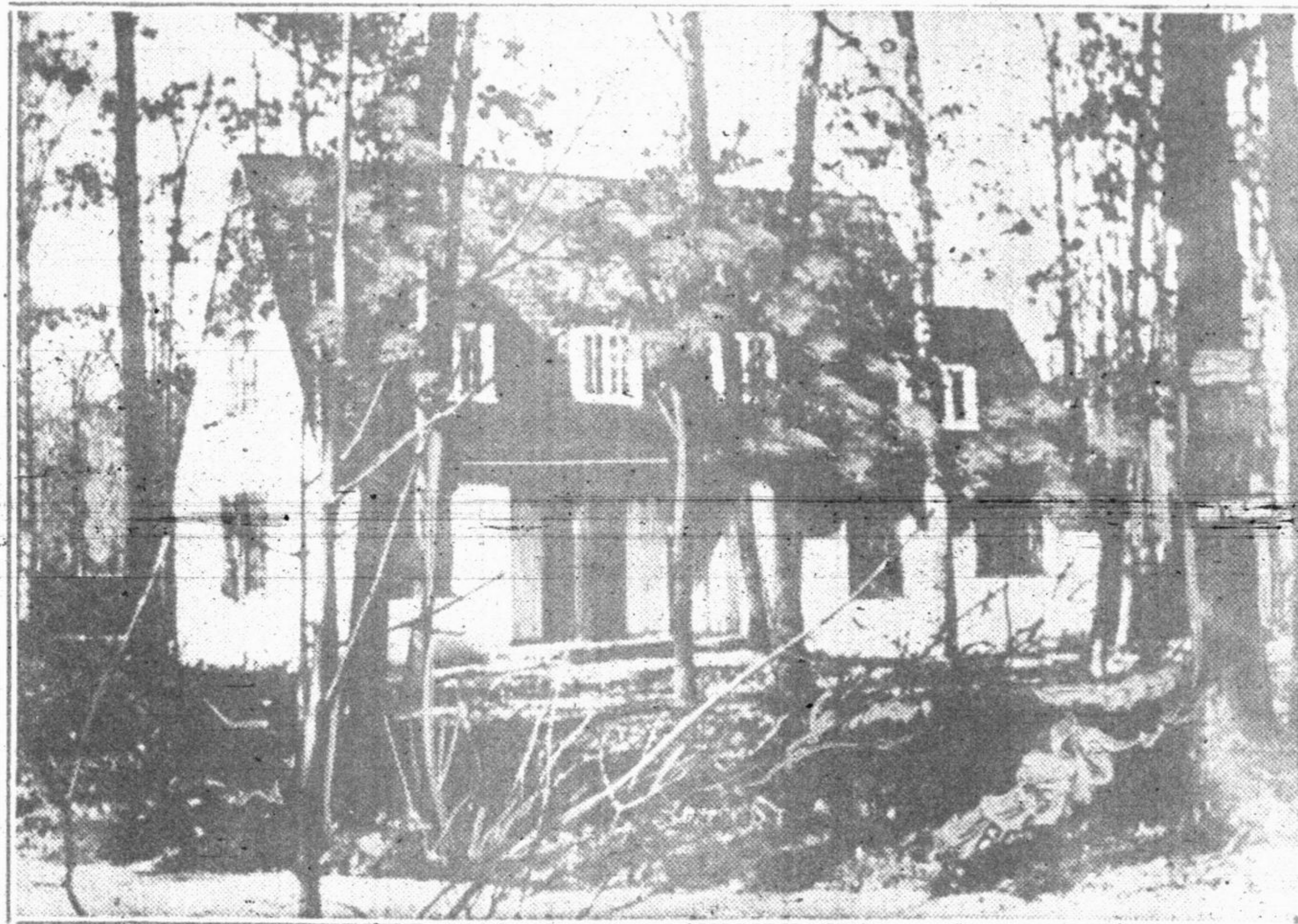
House of English cottage style, built of brick painted white which is situated at 333 Woodland road, Ravinia. This house was awarded first prize in a contest held at the Builders' Exposition of Chicago for the best house costing over $12,000 and under $25,000. The architect is Harry Howe Bentley of Highland Park, whose home is at 337 Woodland road, Ravinia. The cost of the house is reported at $16,500.
