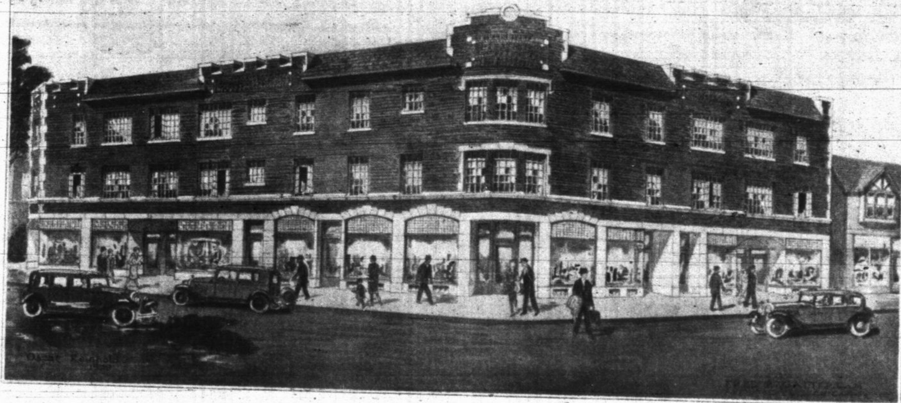
This beautiful building is being erected at the corner of Roger Williams and St. Johns by Mr. Harry J. Luebke. It will have eight stores and fifteen apartments. Earl W. Gsell & Co. has rented the corner store; The J. B. Garnett Co. has rented the east store and the Atlantic & Pacific Tea Co. has taken a store on the Roger Williams side. The stores will be ready for occupancy about May 1st. This is a very marked improvement to the Ravinia business district.
