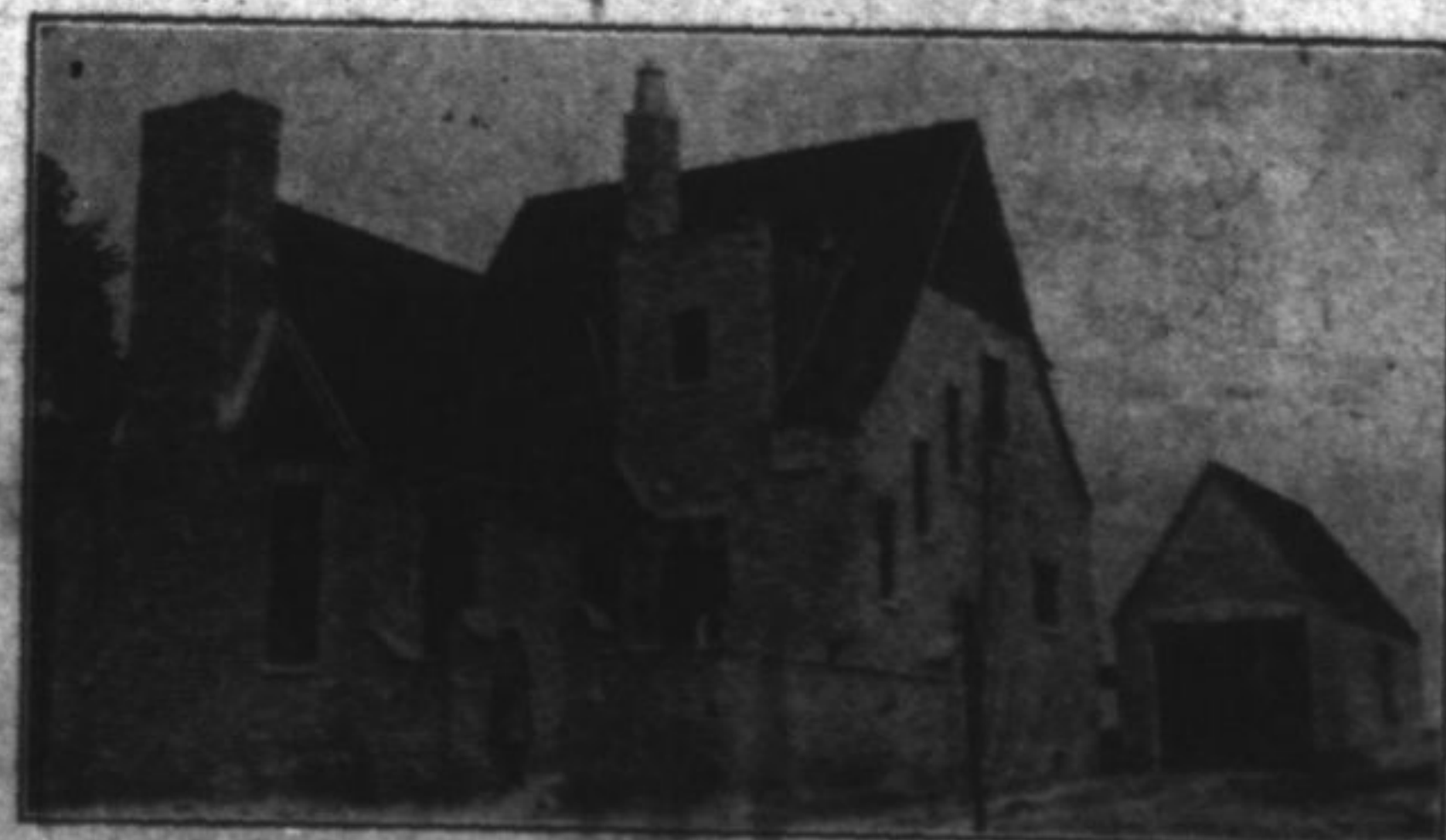
One of the Chicago Tribune prize homes. This beautiful modern five room home was built from a plan submitted by Clarence W. Hunt of New York.
