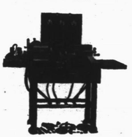
This machine is the last word for testing the electrical apparatus of a motor car. By its use we can quickly and accurately find out what is wrong — and repair it without loss of time.
