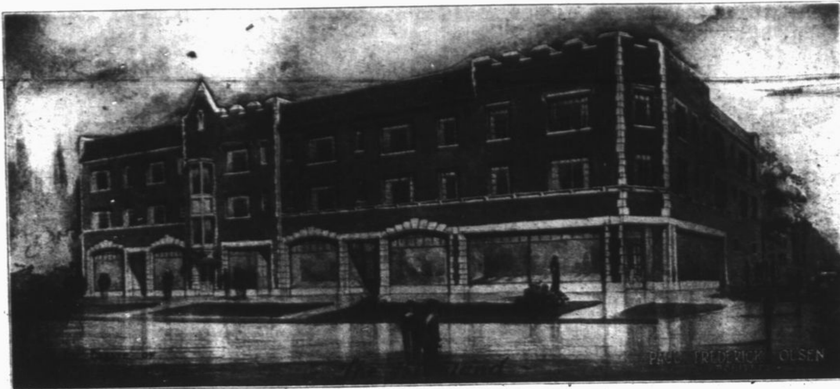
THE HIGHLAND, one of Highland Park's most attractive buildings, being built by Mr. W. H. McKillip, will be ready for occupancy about May 1st. It is three stories high and has six shops on the main floor and sixteen three-room apartments with in-a-door beds and electric refrigeration, some of them so arranged that they may be thrown into suites, and twelve single rooms with bath and maid service. It will probably be furnished by Marshall Field & Co., or Colby & Son. The decorating and interior furnishings will be most attractive. Mr. McKillip will have an office in the building and will have personal charge of the renting.
