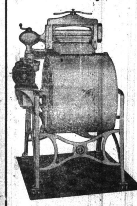
Extra large capacity. Washes 75 to miscellaneous pieces at one time. Does a big washing in one hour. Washes anything that's washable without hand rubbing. Waterproof motor. All working parts completely enclosed prevents accidents.
