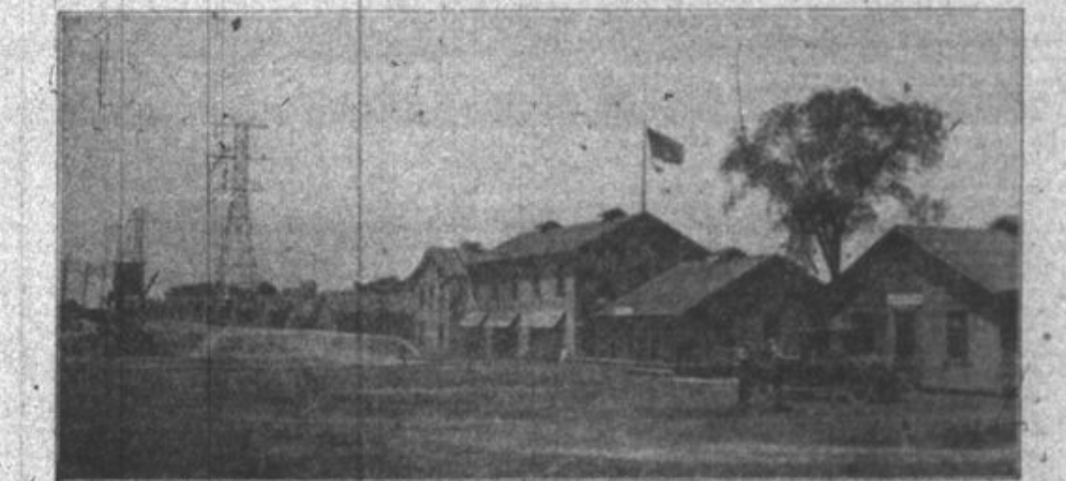
Construction Camp at Blodgett on North Shore Line Branch
