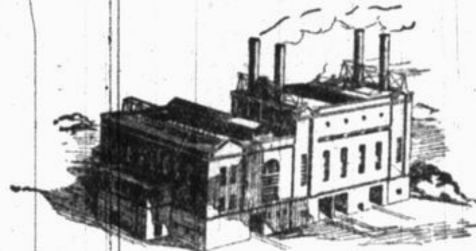
Joliet electric generating station. One of the most efficient in the world. Capacity being doubled.
