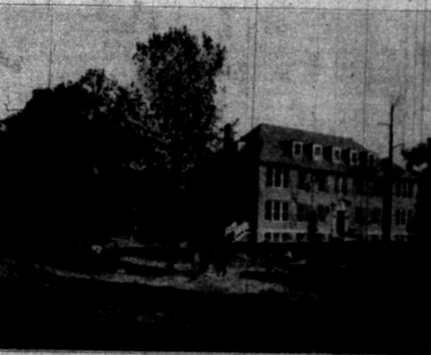
First ground broken for the new wing of the Highland Park hospital.
