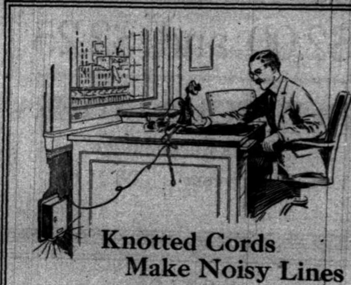
The cloth-covered cord which connects your telephone instrument with the bell box and the cord running to the telephone receiver are each made up of a number of fine wires covered with light insulation. If these cords were not made in this way they would not be flexible. They are necessarily delicate and easily put out of order by misuse.
