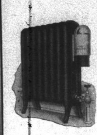
Each "Flobun Humidifier" attached to a Steam or Hot Water Radiator, will evaporate from two to four quarts of water daily-sufficient to moisten the Air in any ordinary room.
