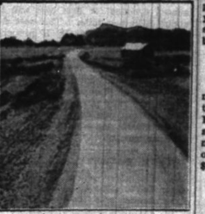
Concrete Road in Mississippi.
