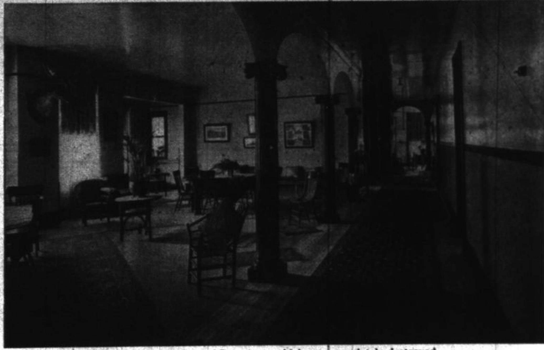
An interior view of dormitory which was completely destroyed
