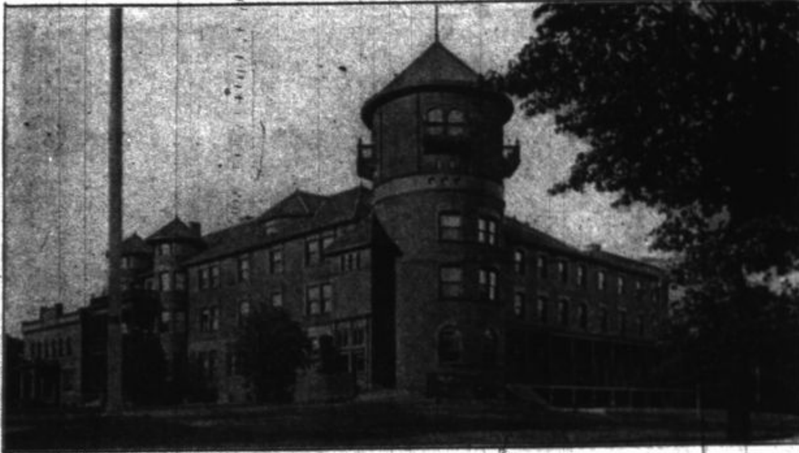
Exterior view of dormitory and mess hall, the latter being saved
