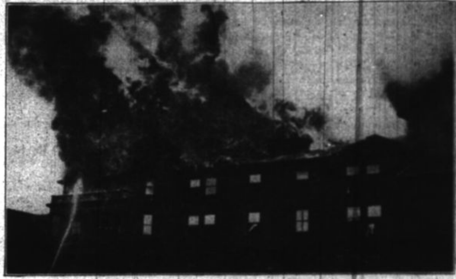
View of Dormitory fifteen minutes after fire was discovered, showing insufficient water pressure. The stream barely reaching the third floor.
