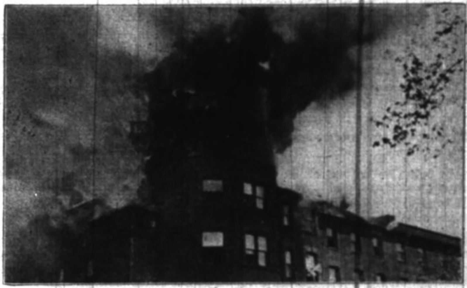
View of tower as fire gains headway
