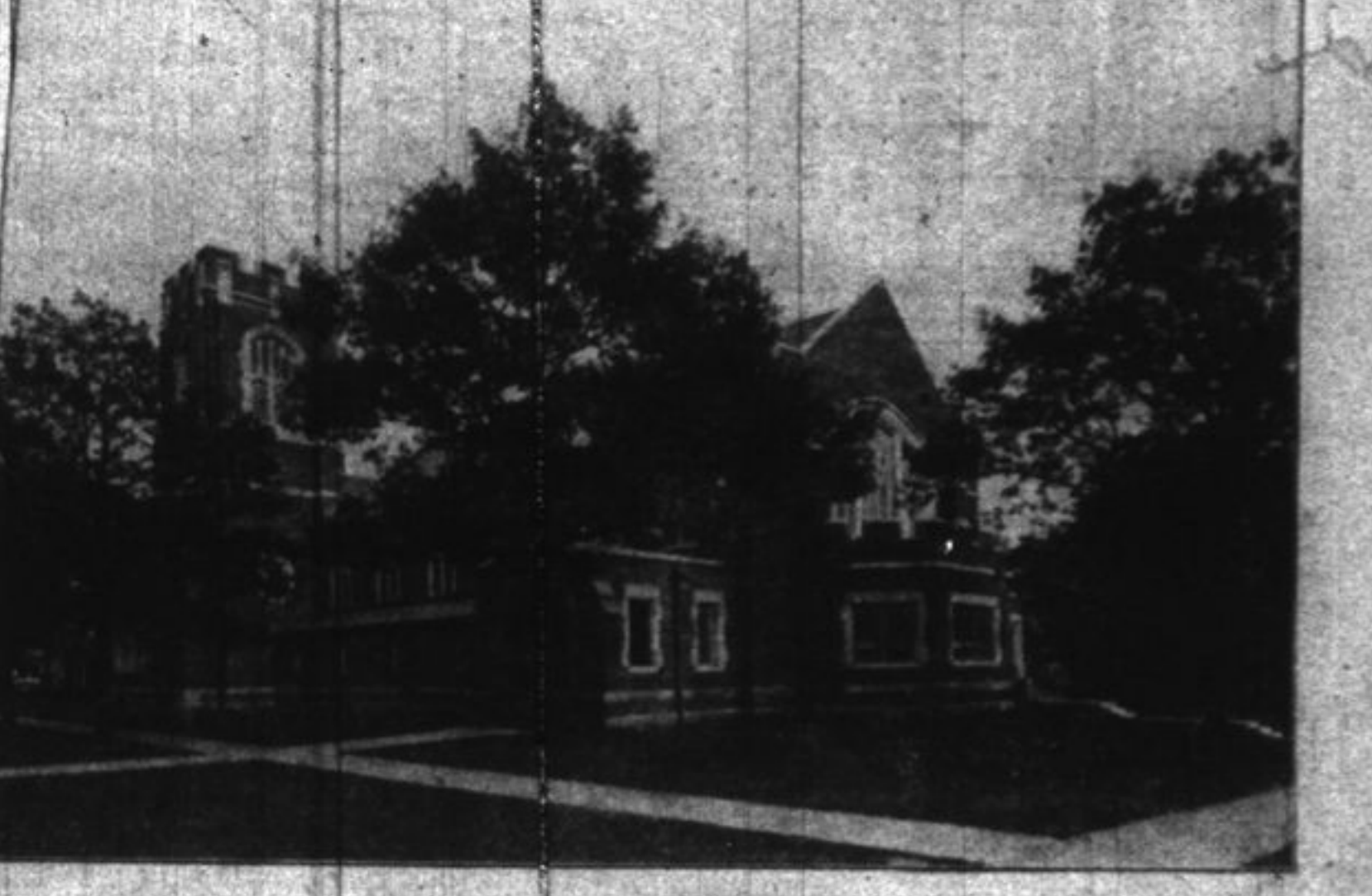
NEW PRESBYTERIAN CHURCH, VIEW FROM WEST SHOWING MAIN ENTRANCE
