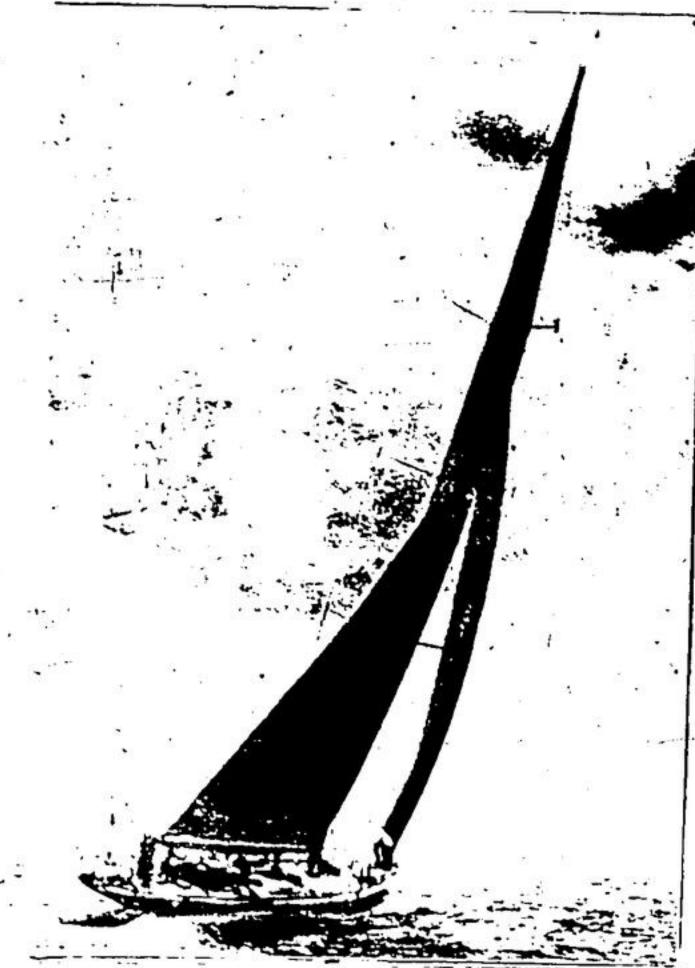
Reconditioned, with new metal must and larger spread of sail, the veteran Yankee clips through the water off Neponset, Mass., in a trial run. The Vankee will compete with the as yet uncompleted Ranger for the honor of meeting T. O. M. Sopwith's Endeavor II., for the America's cup Gerald Lumbert owns the Yankee.
