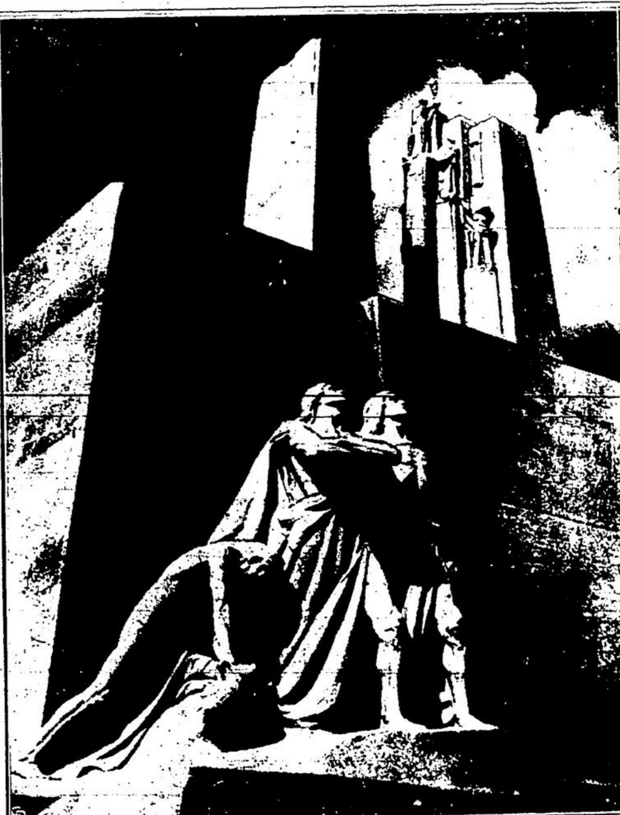
Here is an impressive view of Canada's on July 26th. Erected to perpetuate $11,250,000. Thousands of Canadian war veterans will pilgrimage to Vimy next month to witness the unveiling, which will be unveiled by King Edward taken 11 years to complete, and has cost
