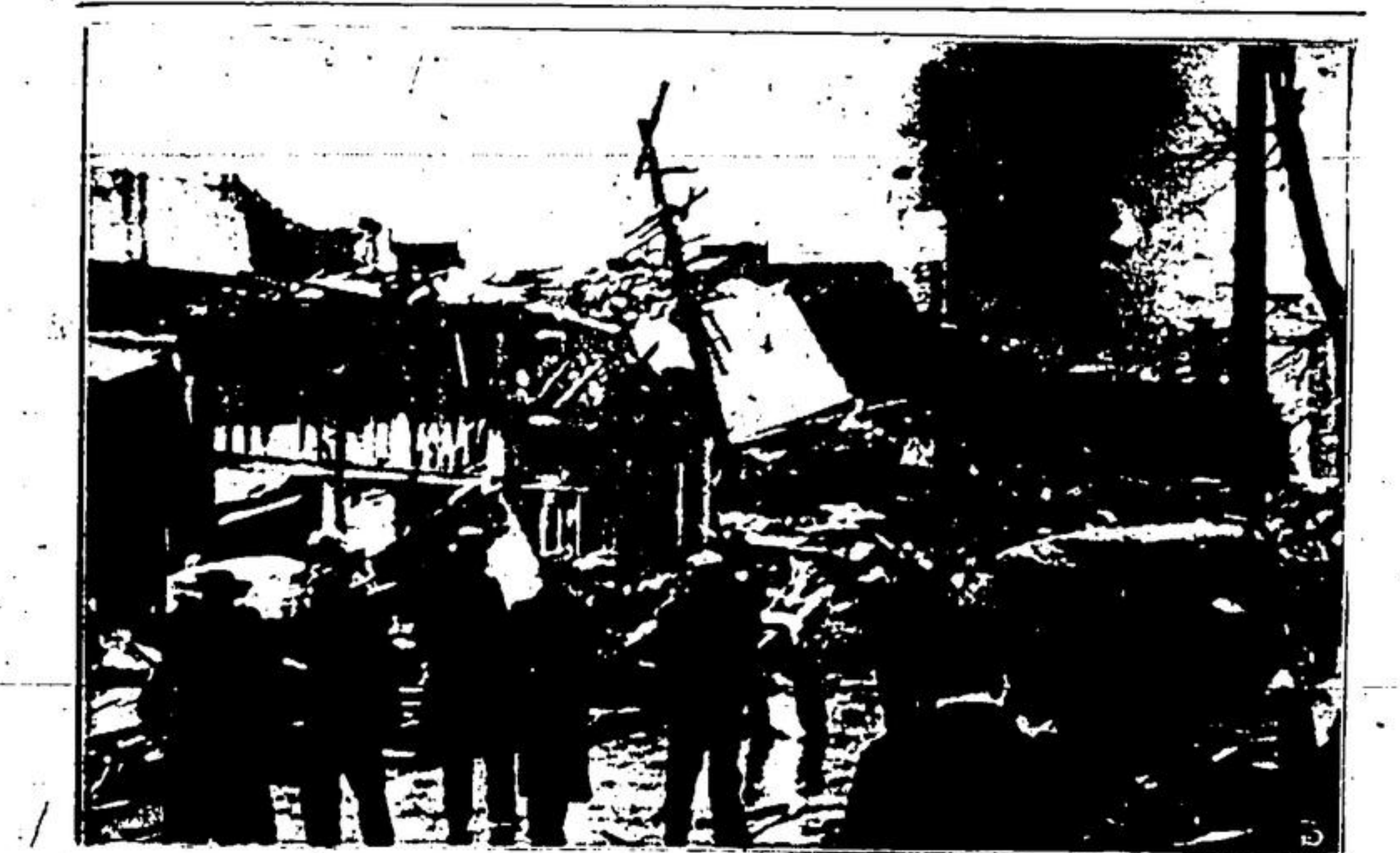
Broken gas mains, and electric their lives in the wind storm; and 1,000 more were injured. Property damage, that was greatly increased by the fires, will probably reach $5,000,000. This picture shows a ground.
