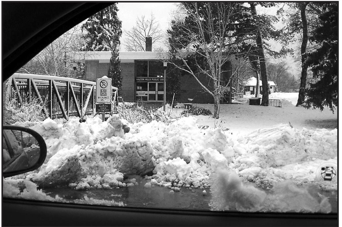
NO STOPPING: Acton branch of Halton Hills Library is always a picturesque spot in all seasons but it gains a postcard look when snow falls. The Bailey bridge which spans the School Creek, heavy with frost, nevertheless presents a unique entrance to the yellow brick building, good for a photo from a car window.
