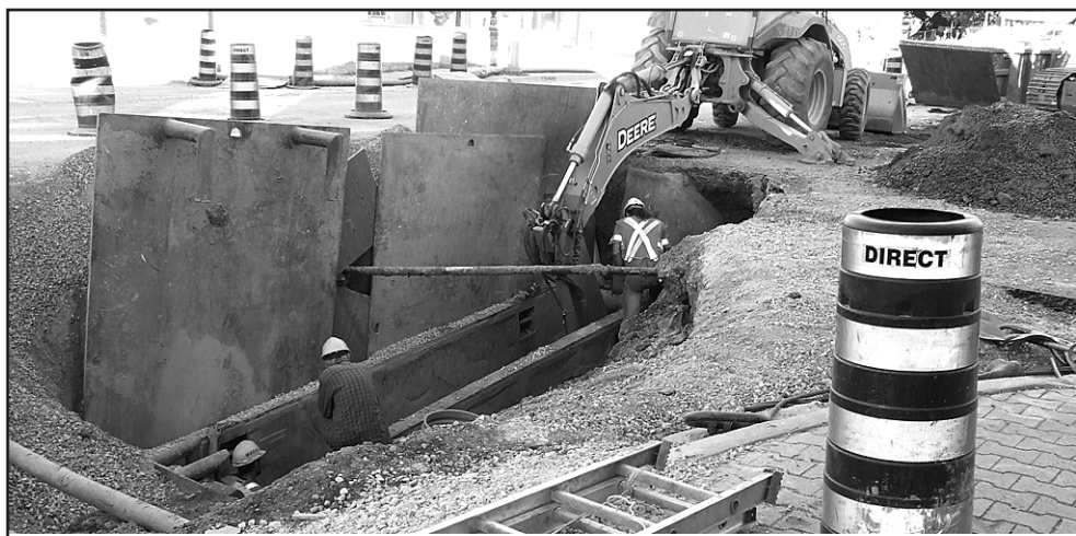
Workers dig deep under Main St. to install sewers, watermains.
