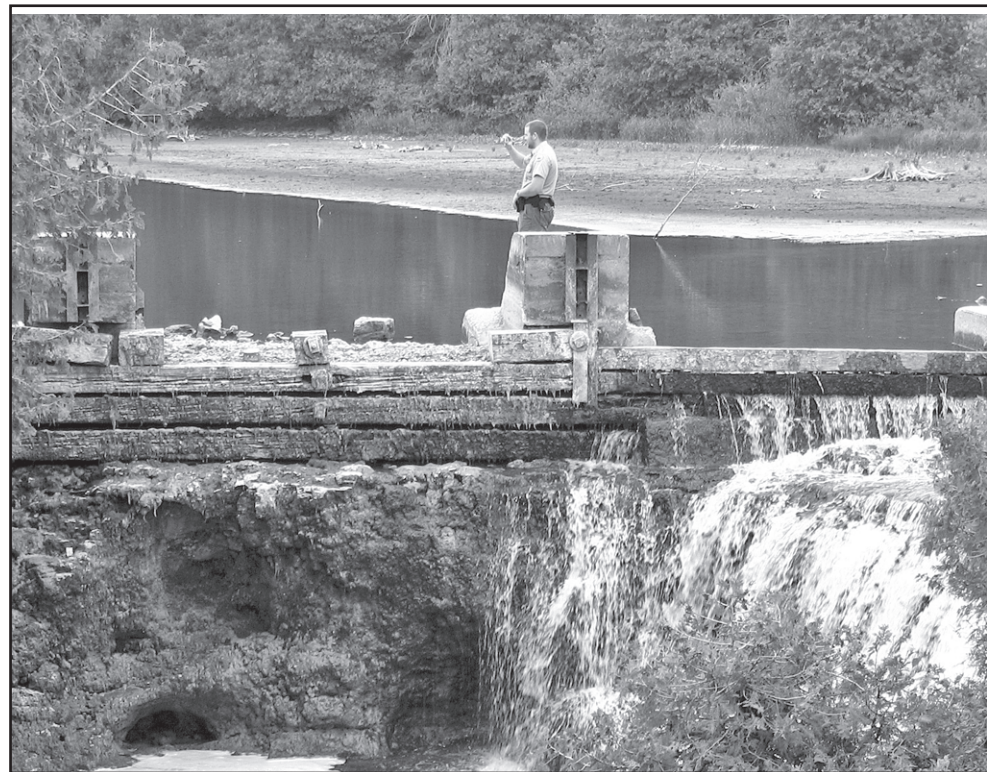
LET IT FLOW: The Grand River Conservation Authority decommissioned the upper dam in Rockwood this spring to "renaturalize" the river. Better flow should lower water temperatures and improve water quality. Shown here, a staff member takes photos of the river and shore to document its progress. Rebecca Ring Photo
