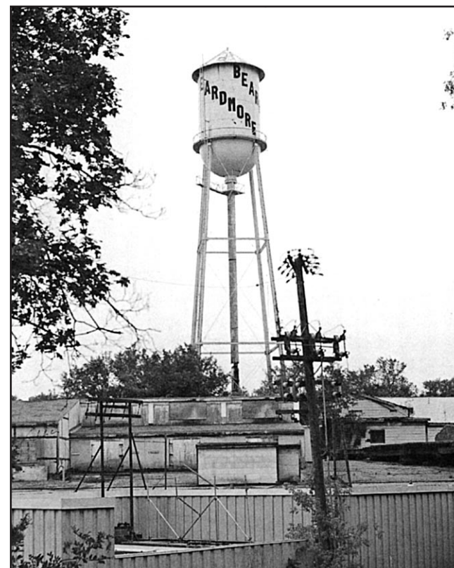
The Beardmore water tower stood like a sentinel over the huge complex until it was taken down in 1999.
