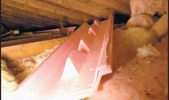
*Install styrofoam deflectors to prevent the insulation from obstructing the air vents.*
