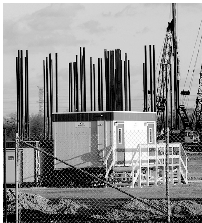
An artist's rendering of TransCanada Energy's 683-megawatt natural gas-fired power plant on Steeles Avenue and Sixth Line South in Hornby. (Below) Steel beams, or piles, for the plant's frame have been installed in recent days.
